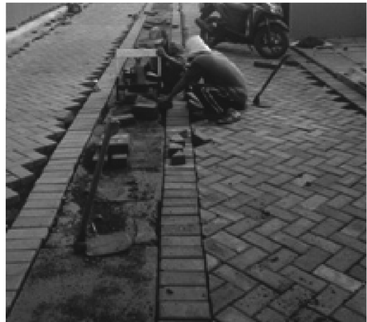
Sumber: www.cv-aditirtaaspalhotmix.blogspot.com Gambar 3.24 Tukang sedang memasang paving
