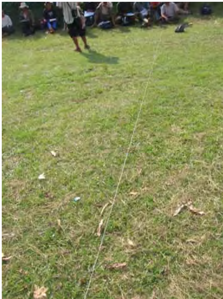
Gambar 184. Menarik garis as reaktor biogas
