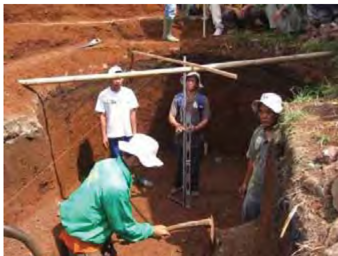
Gambar 44. Pemasangan tiang as
