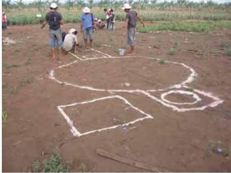
Gambar 191. Gambar lay out galian reaktor biogas
