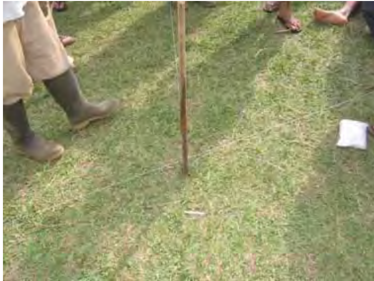
Gambar 185. Menentukan as tangki pencerna
