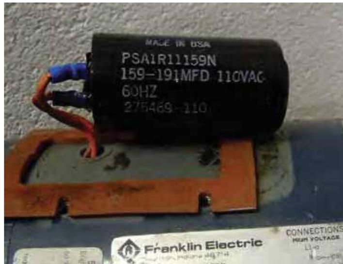
Gambar 5.3 Tipikal Starting Capacitor (159-191 mfd)
