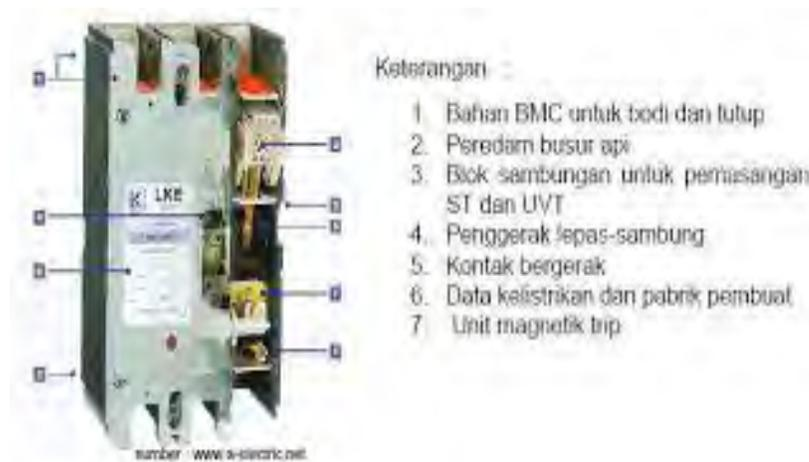
Gambar 2.22. Moulded Case Circuit Breaker
